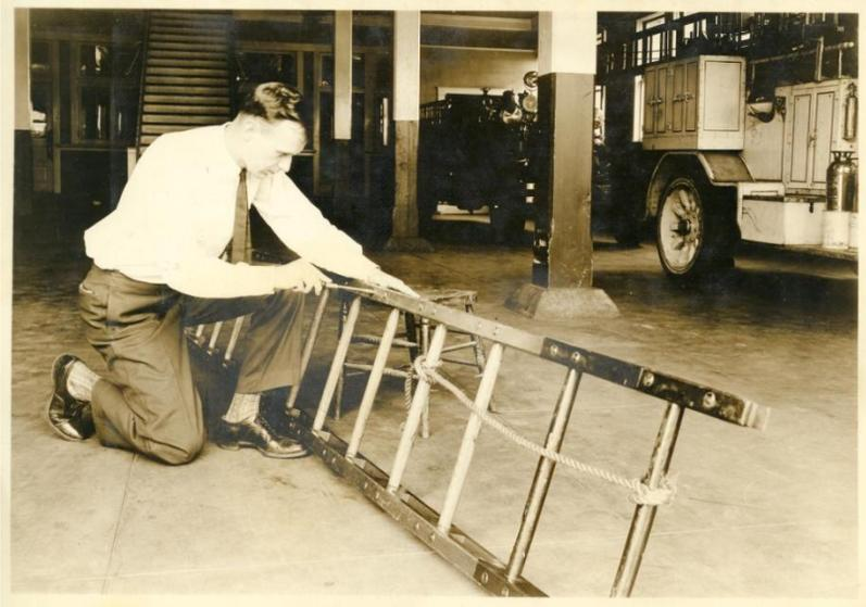
coating. When necessary, the old finish would be scraped off, the ladders sanded, and then re-coated with gym seal. This might occur several times a year for busy companies. The relative age or experience of wooden ladders could often be measured by how rounded the corners would be from the re-finishing process.
