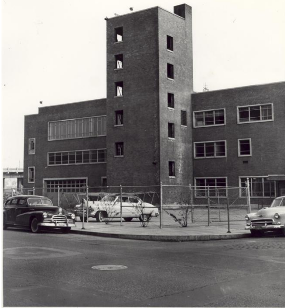
1950 Station 1 Drill Tower
