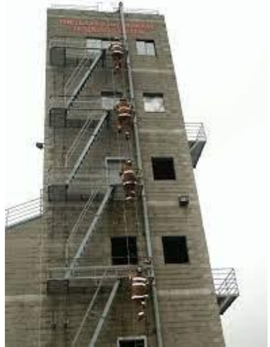
Station 2 Drill Tower
