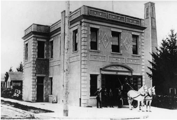
Built 1913 - Station 30 8105 N Brandon Avenue
