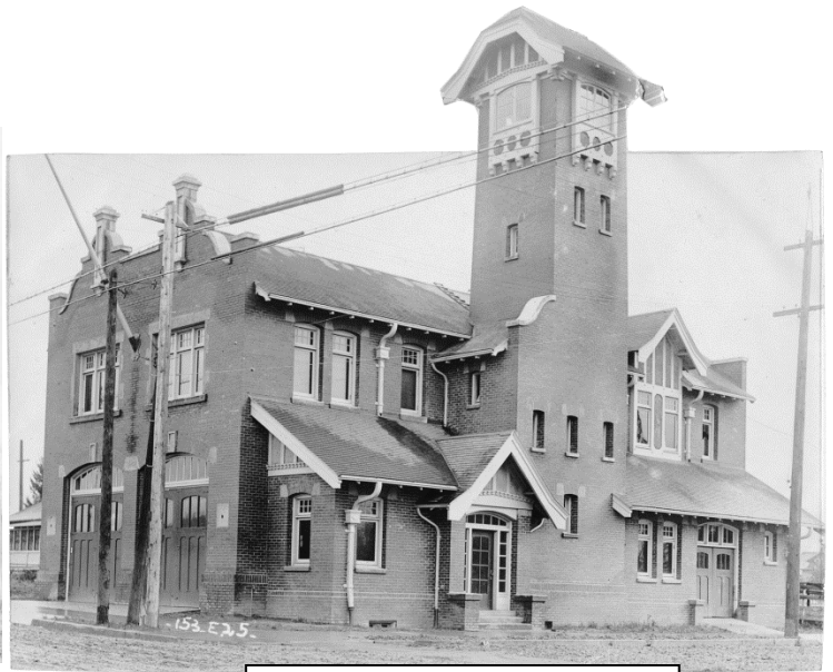
Built 1912 - Station 25 3350 SE Francis Street
