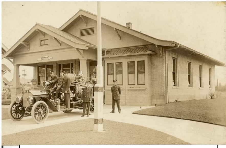
Built 1913 - Station 18 2200 NE 24th Avenue - Prototype Bungalow Station
