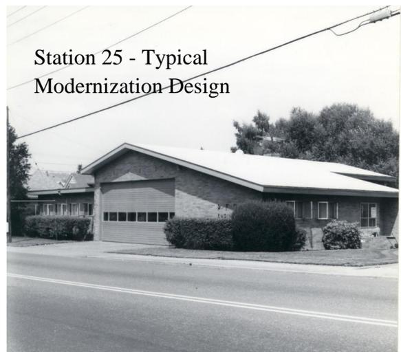
8,000 per station, and to present less objectionable building lines in residential neighborhoods. Fire hose will be dried in electric hose dryers and stored in portable hose racks. The roof is a 20 year roof with 1 ½ inch insulation to retain heat in the building. Heat is by hot water with the building divided into four zones or areas.
