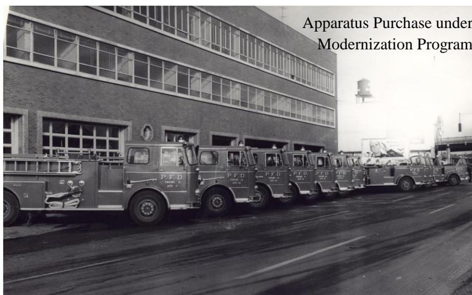
vision. The apparatus provides seats for five men. Each new apparatus is equipped with 100 ampere alternators, wired for "plug-in" cords to supply flood lights or other electrical equipment directly from the vehicle engine. Self contained gasmasks are carried on all this apparatus.
