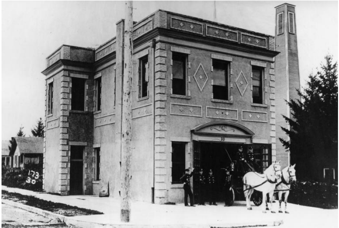
Built 1913 - Station 30 8105 N Brandon Avenue
