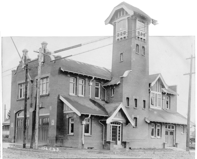
Built 1912 - Station 25 3350 SE Francis Street
