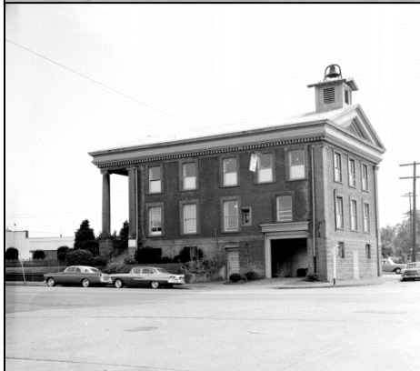
A side view, showing the apparatus door to the basement fire station.
