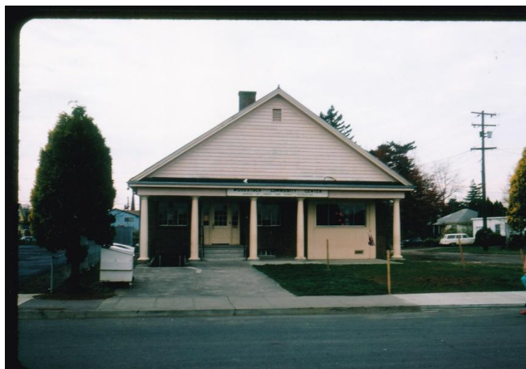
Built 1928 - Station 11 5905 SE 43rd Avenue
