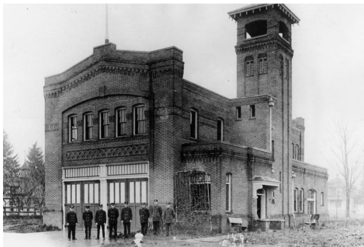
Built 1911 - Station 24 5340 N. Interstate Avenue
